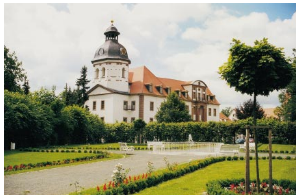
Christiansburg with the palace gardens and church. This magnificently ornamented building is considered to be the most remarkable baroque church in Thüringen.
